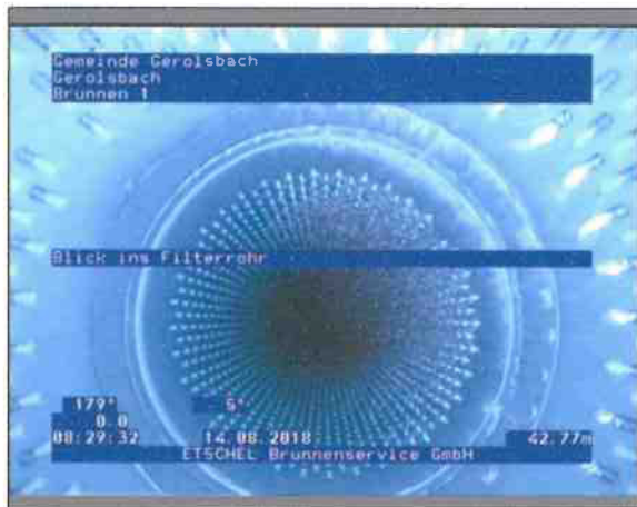
Foto: 1_1_12_14082018_082754_A.JPG 42,77m, Blick ins Filterrohr
