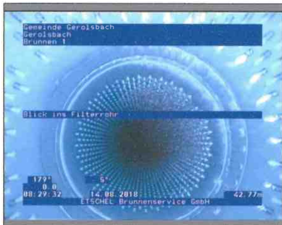
Foto: 1_1_12_14082018_082754_A.JPG 42,77m, Blick ins Filterrohr
