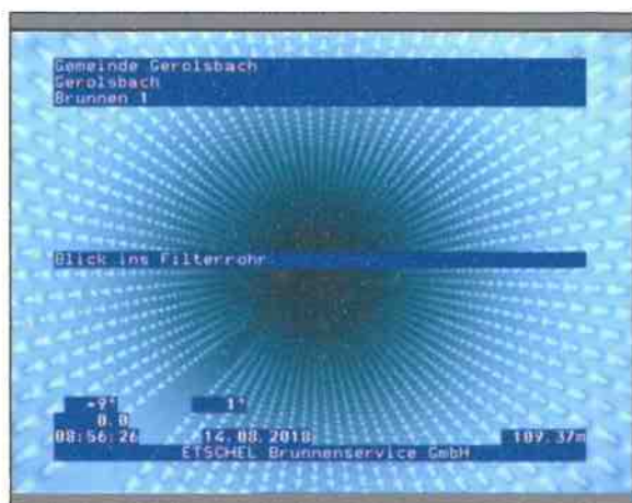
Foto: 1_1_25_14082018_085447_A.JPG 109,37m, Blick ins Filterrohr
